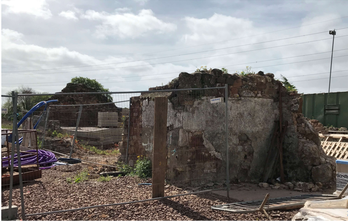
Figure (ix) Looking East Towards the Existing Building.
