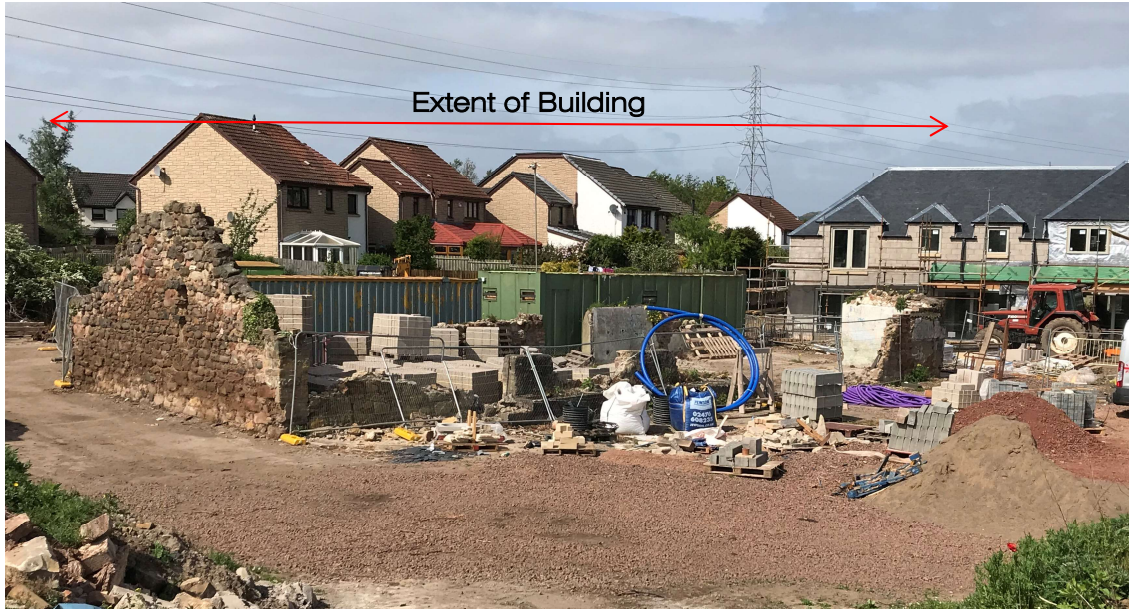
Figure (vii) Existing Building Looking South-west.
