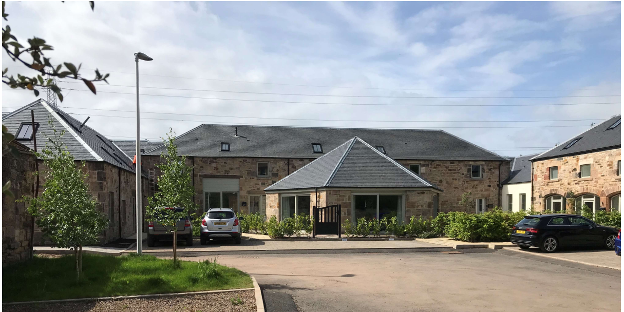
Figure (v) View of Brunstane Steading Phase 2 Courtyard Looking South.
