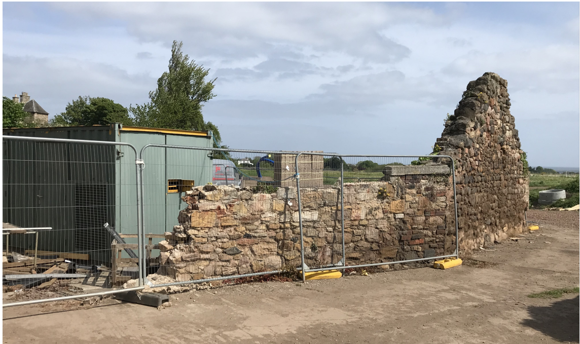
Figure (viii) Looking North Towards the Existing Building.
